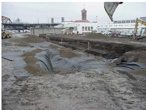
FIGURE 1. Lots 1 and 2 at beginning of construction.
